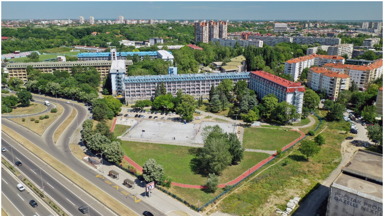
Figure 24 The zone of new construction
