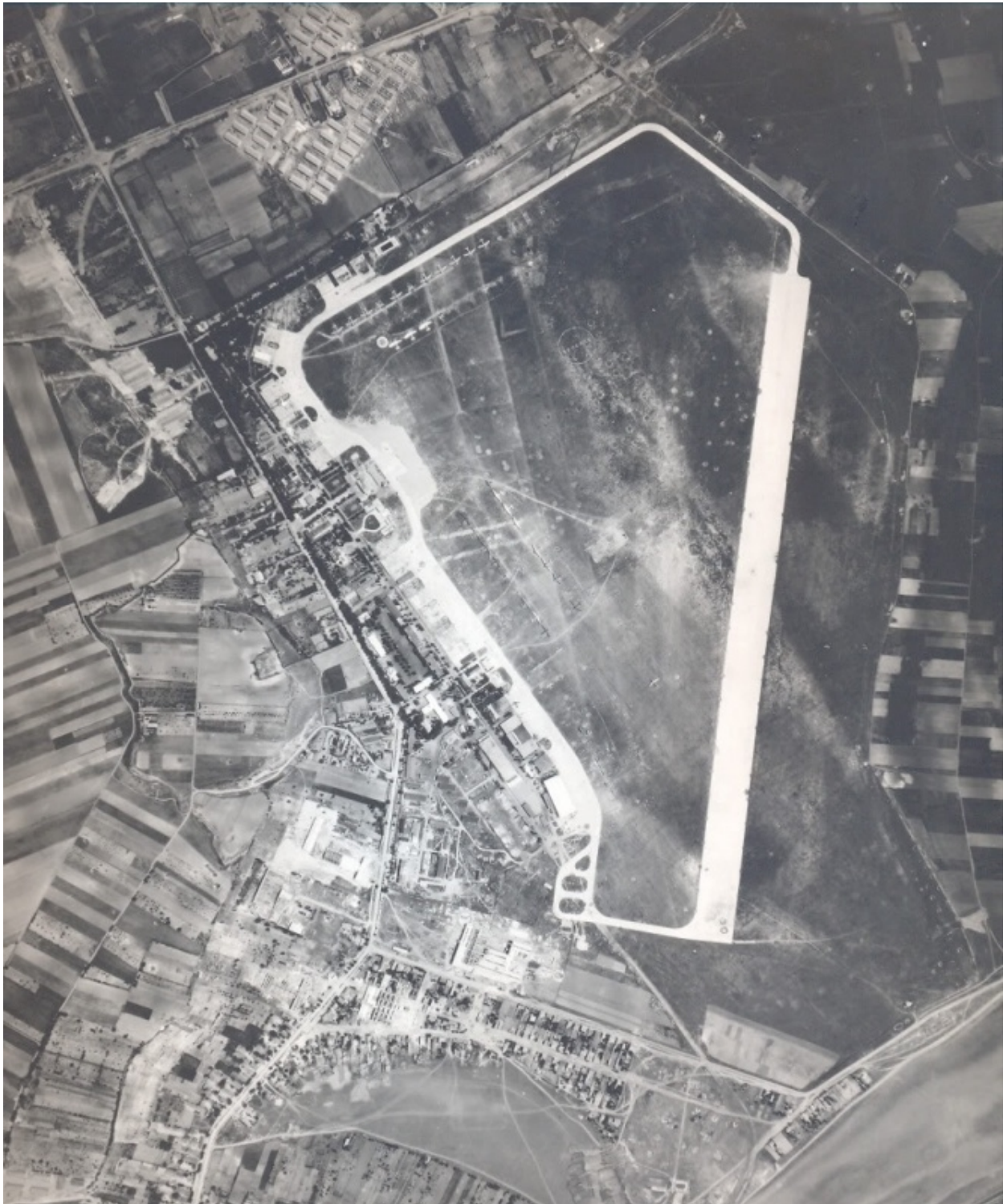
Figure 11 Old Belgrade Airport, immediately before the Second World War
